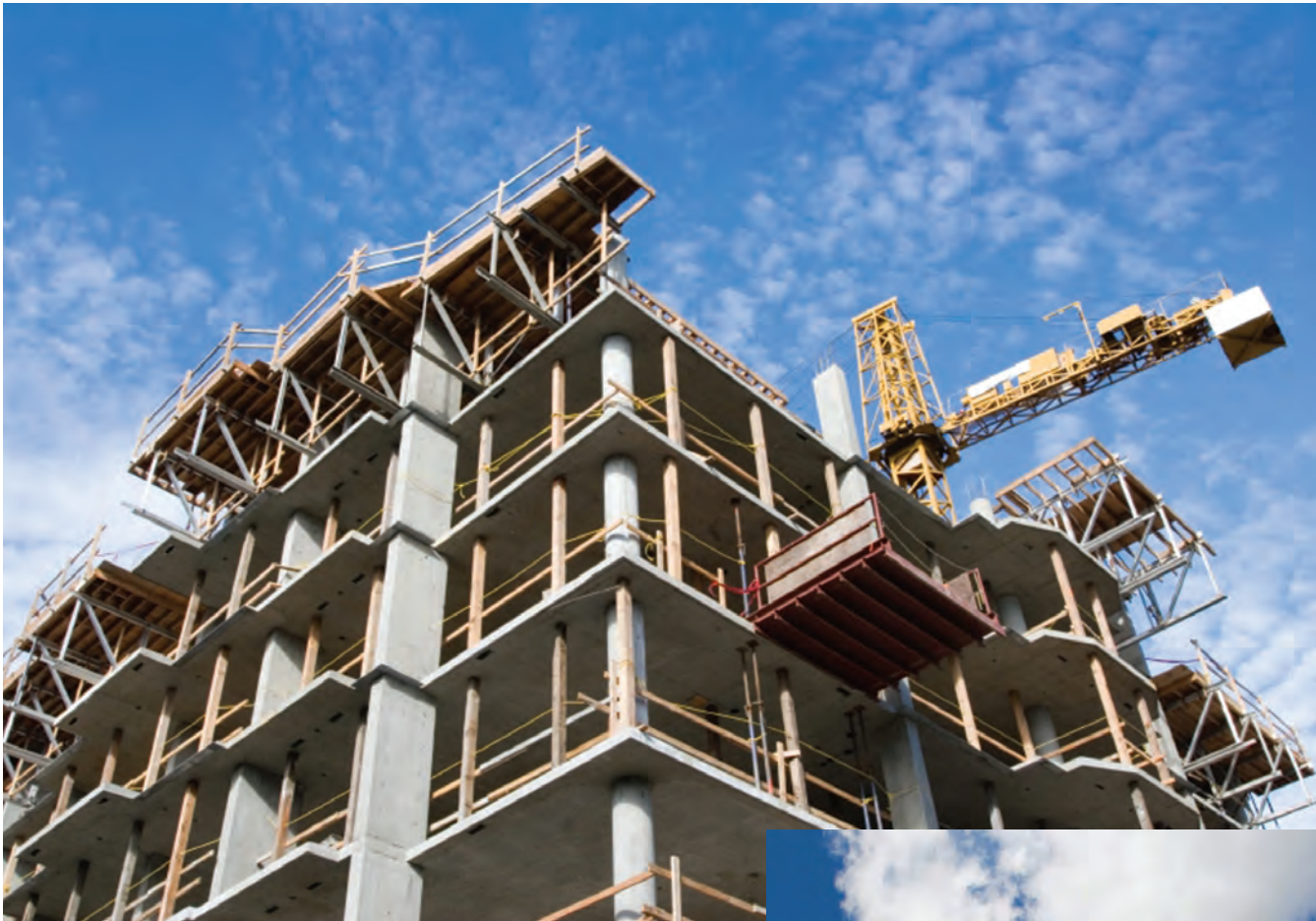
Construction Elevator Emergency Stops
