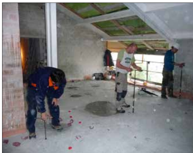
Installation of an FZH+Sylomer® floor mount.
