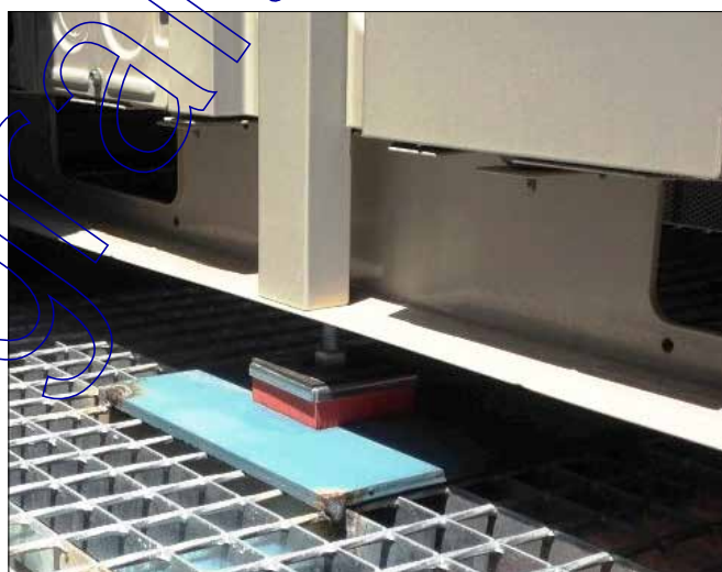
Example of installtion of a TSR+Sylomer®
