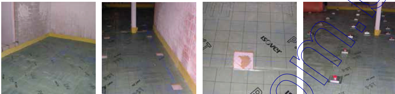
Conditioning the premise and installation of the mounts.
